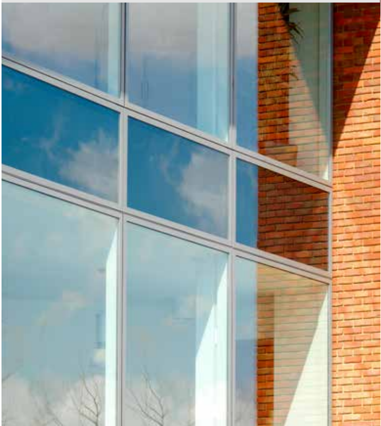
FAÇADE WITH VELFAC 200 WINDOWS AND RAINSCREEN PANELS
