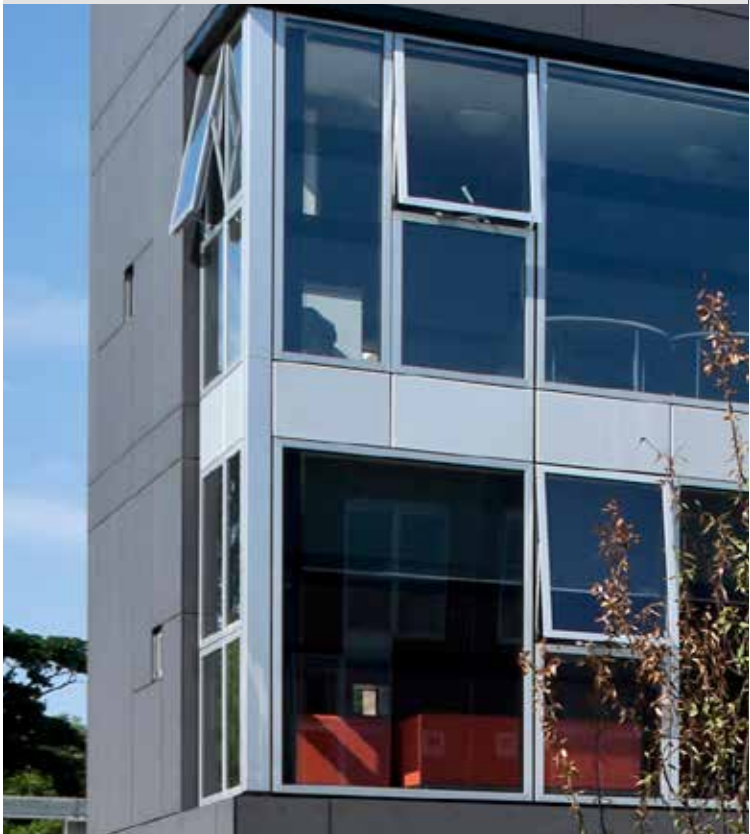
FAÇADE WITH VELFAC 200 WINDOWS AND RAINSCREEN PANELS
